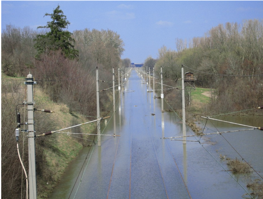
Flooding, March flatlands, 2006
